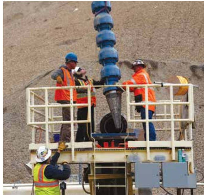
Goulds vertical turbine being installed for a mining application.
