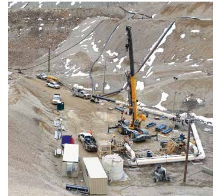
Pumping system installation for leaching at a gold mine.
