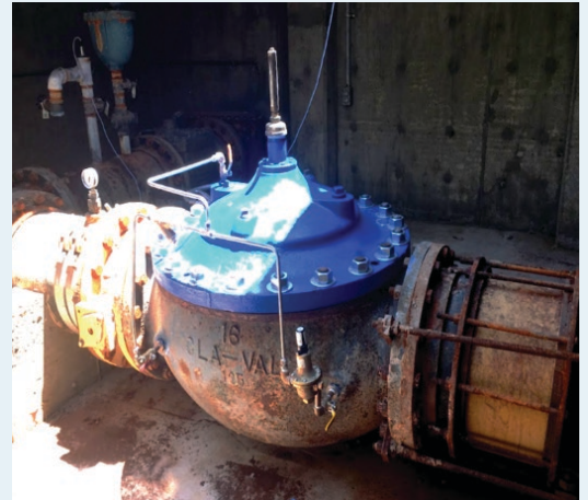
An example of a large water distribution Pressure Reduction Valve (PRV) installation
