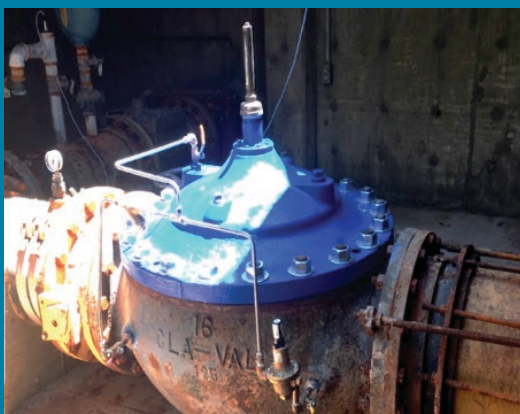
Pressure reduction valve
