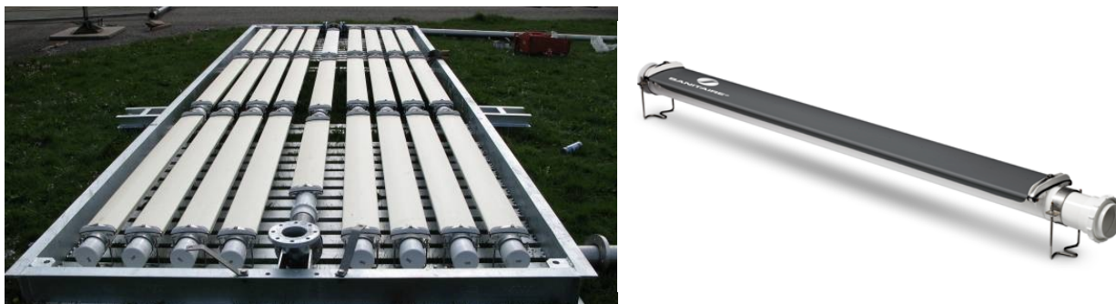
Figure 7. Left: example of an installation of Sanitaire (a Xylem brand) Gold Series HDLF diffusers on a liftable grid with a 40% diffuser density. Right: single Gold Series diffuser.
