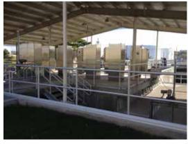
Stainless steel air conditioned ballast cabinets supply the power to the UV lamps
