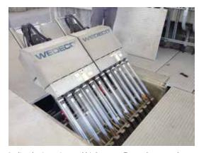
Inclined orientation and high power Ecoray lamps make for a small footprint, reducing construction costs
