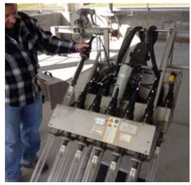
The automated lift and modular design makes maintenance quick, easy and safe.
