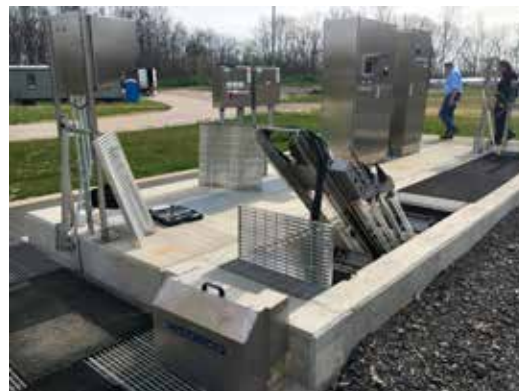
Weather proof stainless steel cabinets protect UV electrical systems and controls
