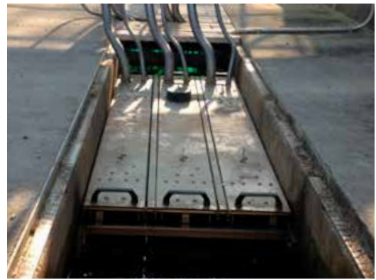
Installed Wedeco UV solution.
