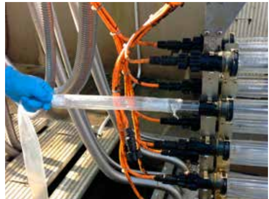
Changing a lamp in a Wedeco UV module.
