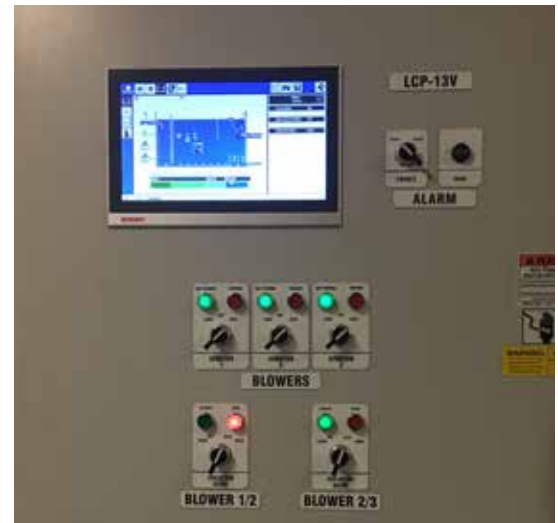
Updated HMI hardware and software includes larger screen and more intuitive graphics
