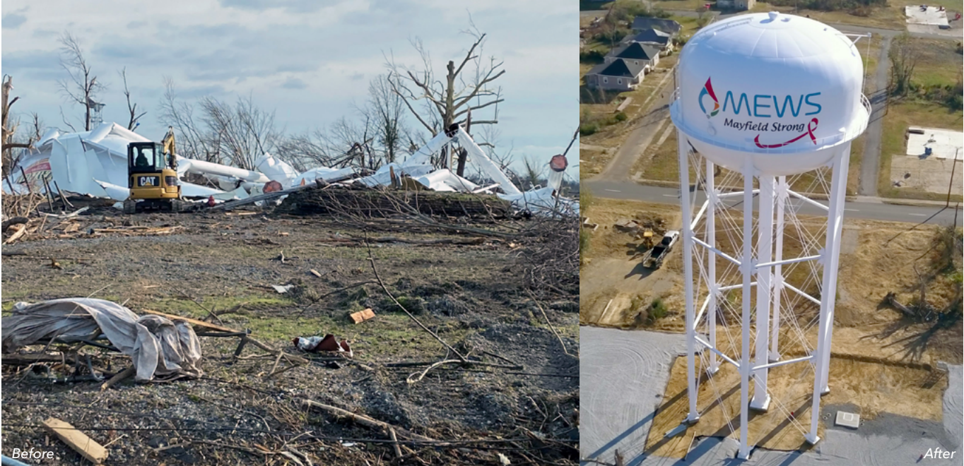
The tornado completely destroyed Mayfield's 600,000-gallon elevated water tank, but a new one stands in its place with the spirited tagline "Mayfield Strong" as the community continues to rebuild.
