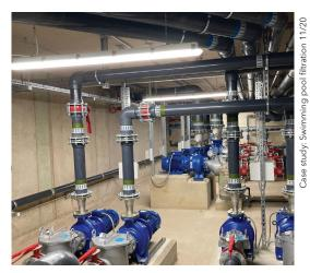
New design, high-efficiency Lowara e-NSC series circulation and feature pumps for the main pool and leisure pool at Braywick Leisure Centre.
