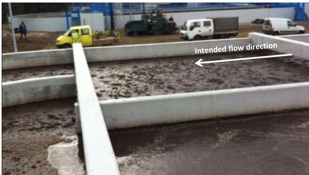
*Figure 1. Back flow hinders floating sludge from passing through the bend at Tata WWTP, Hungary.*
