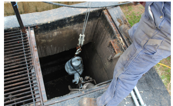
The Concertor pump is lowered into position.
