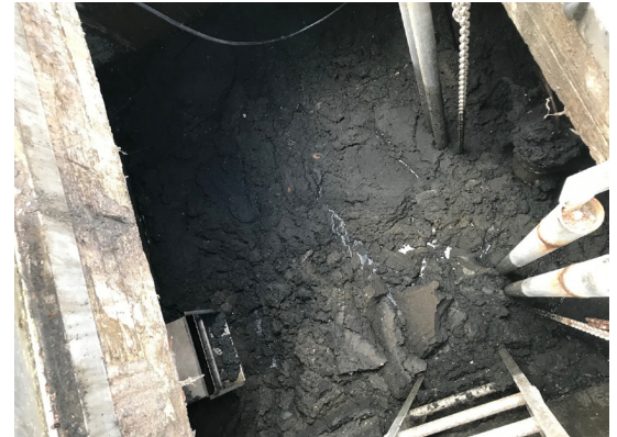
High levels of debris and grease accumulation once plagued the Cowansville pump station.
