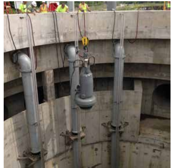
Flygt model CP3351/995 FM 800 HP 4160V, 10417 gpm at 192' tdh
