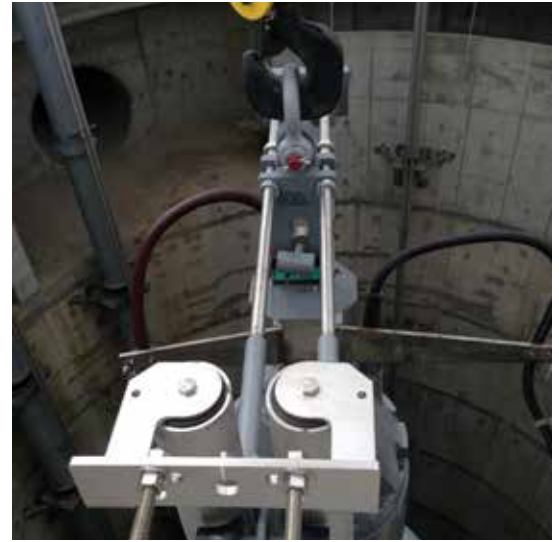
Flygt pump being installed on guide rails
