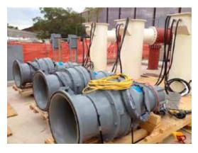
Flygt pumps ready for installation at the Chihuahuita Storm Sewer Pump Station
