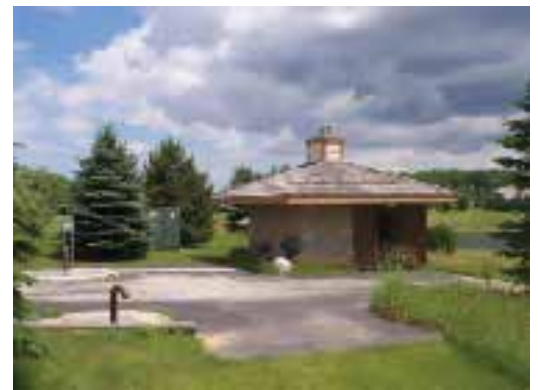
A lift station in the village of Hartland, WI
