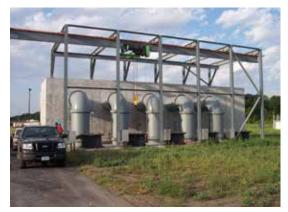
A worker shown in context with massive elbow bends at the discharge lines for the array of five, 100-mgd, 640-hp direct-drive Model PL7121 pumps supplied by Xylem's Flygt team. The massive units resolved effluent blockages once induced by high flows down the Missouri River.
