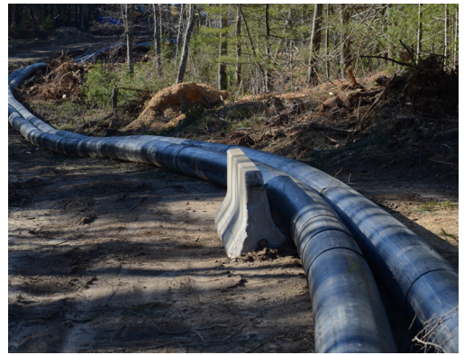
The two miles of HDPE pipe had to be fused 500 feet at a time at the work area and then dragged through the woods and over rigorous terrain to get to the break.
