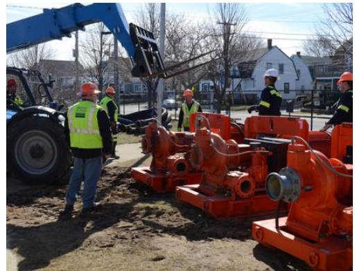
Four Godwin HL200 pumps were brought in to override the pumps at the Water Street Pump Station.
