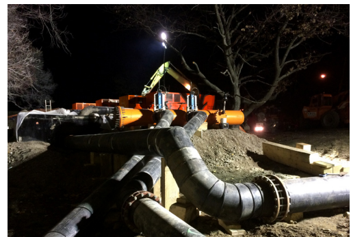
Night work: 18-inch bypass lines coming off the manifold with four Godwin pumps in the background.
