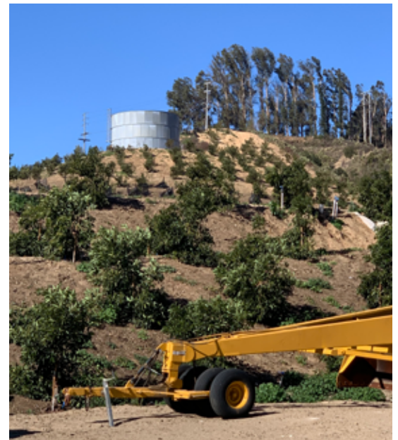
Installing the IPC in the NEMA 3R enclosure helped protect Eat Sweet Farm's irrigation system in its remote location.
