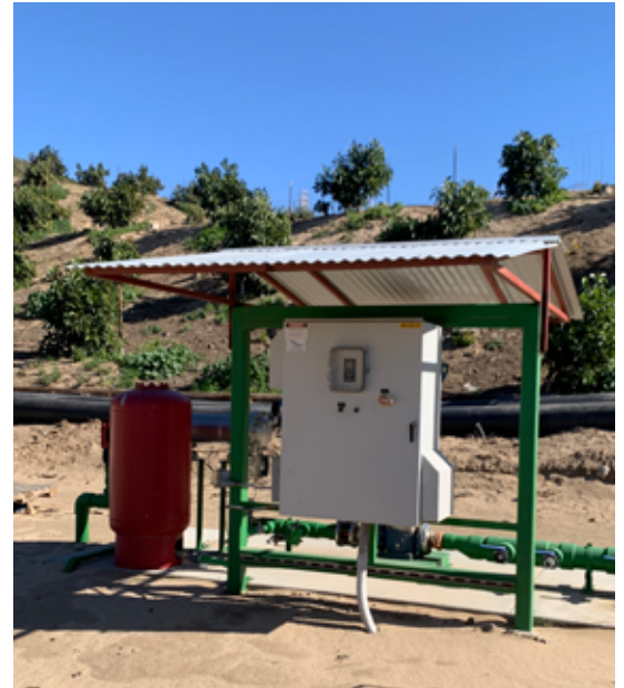
For outdoor applications, it's important that the VFD system is protected from exposure to weather, dust, heat or other environmental factors.
