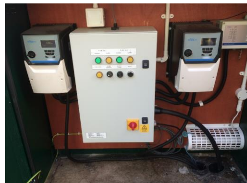
Above: Compact space saving control panel design with SmartRun pump controllers.
