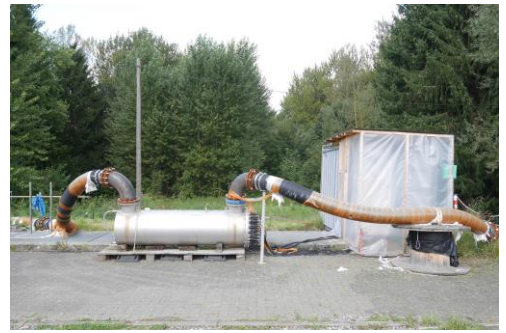
The LBX UV system was addressing the Legionella issue instantly and treated the effluent effectively for one year. With the rental service the operators gained time to find an appropriate permanent solution.
