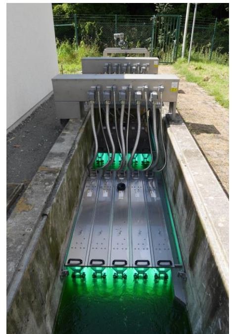
Warstein awarded Wedeco with the supply of a permanent disinfection solution. The Wedeco TAK 55 UV disinfection system was installed in August 2014, delivering safe wastewater requiring minimal energy and ultimately improving water quality in the River Wester.
