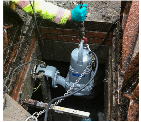
Installation of Flygt Concertor at Yorkshire Water's Burnsall Car Park site.
