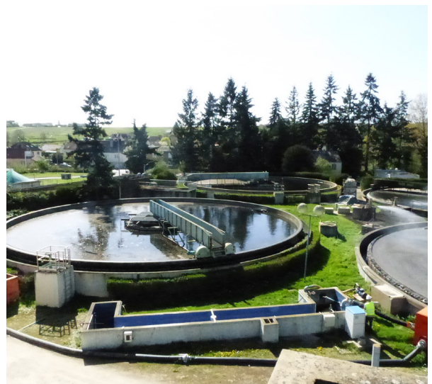
The old treatment plant at Lèves, before construction of the new plant began at Mainvilliers
