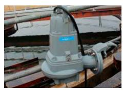
Concertor® pump being removed after 1 month of operation for inspection.
