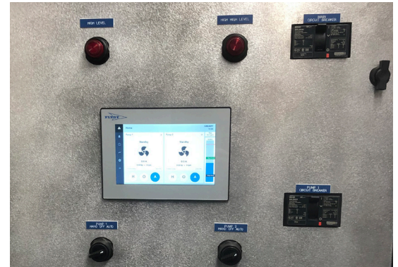
The compact Concertor XPC control panel with intuitive touchscreen controls.
