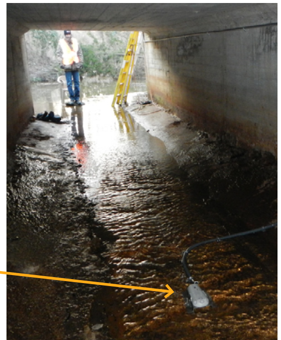
SonTek IQ Acoustic Doppler Profiler based open channel/non-full pipe flow meter being installed in a typical stormwater culvert.
