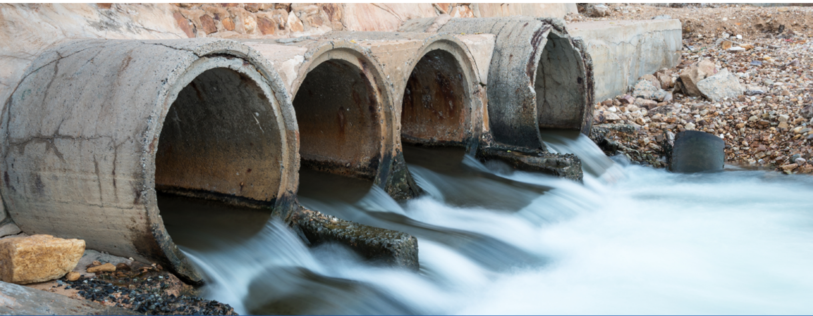
Storm drain outflows
