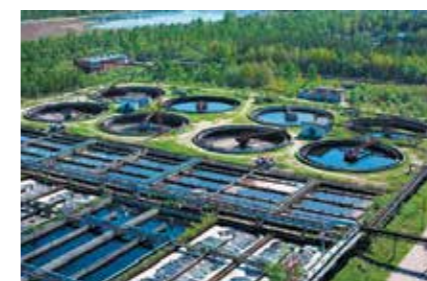
Municipal Wastewater Pumping & Treatment
