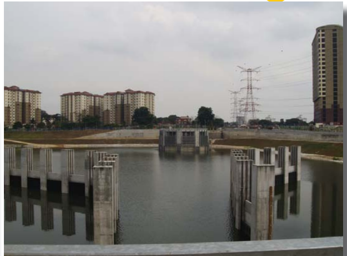
Intakes for the SMART system can draw millions of cubic meters of floodwater into a massive underground tunnel, sparing the streets above from crippling floods.
