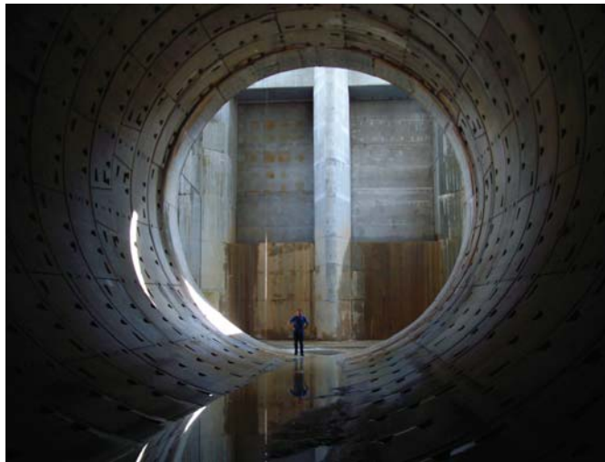
At 11.8 meters in diameter and 12 km in length, Kuala Lumpur's SMART tunnel and its associated holding ponds can capture up to 4 million cubic meters of floodwater and divert it away from flood-prone downtown.
