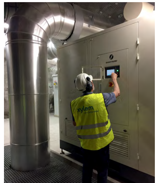
Xylem employee assisting in startup of TurboMAX 600 (400kW) blower.
