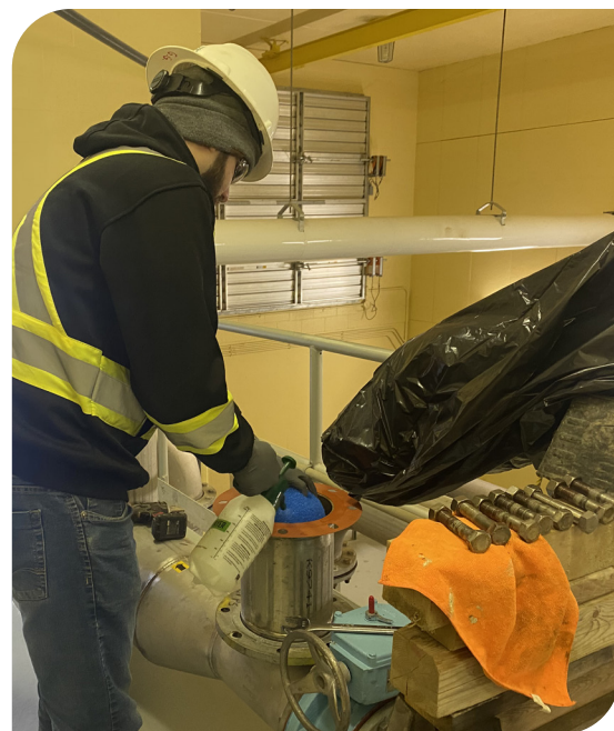
SmartBall insertion at the pump station
