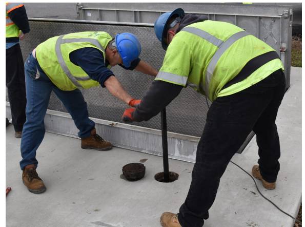
Valve condition assessment
