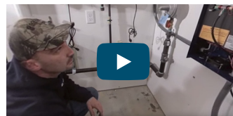
Goulds Water Technology Submersible Pump Installation (360 Video)
