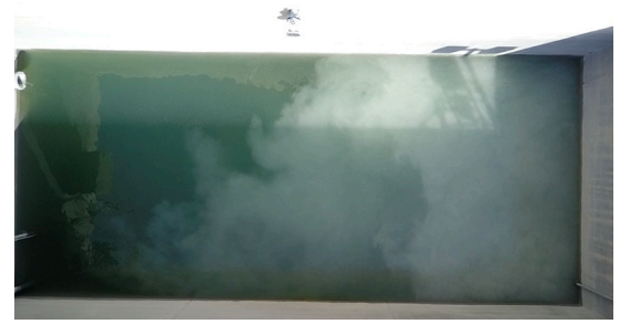
Lime sludge being resuspended by Flygt Adaptive mixer.
