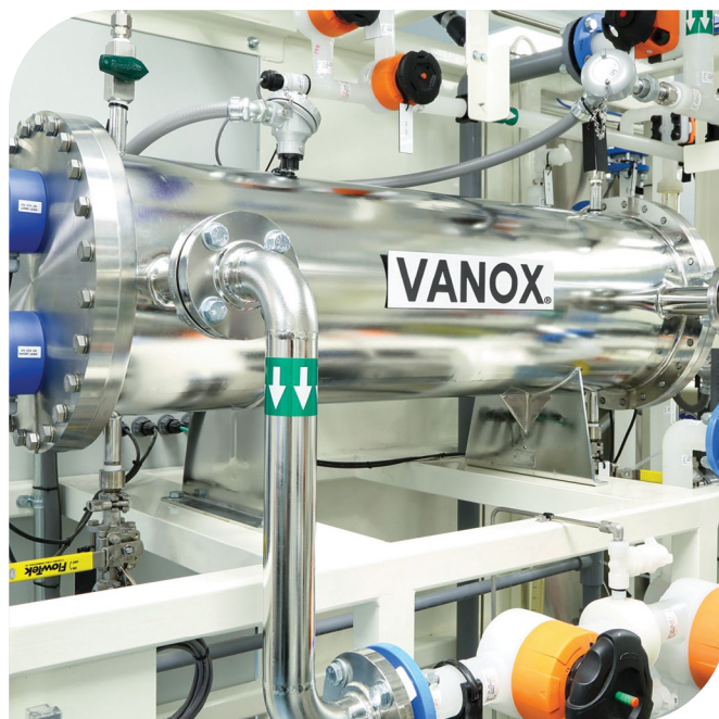
AOP reactor within the Vanox® POU system
