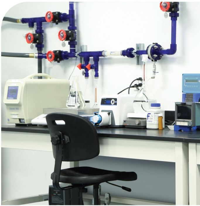
TOC injection station
