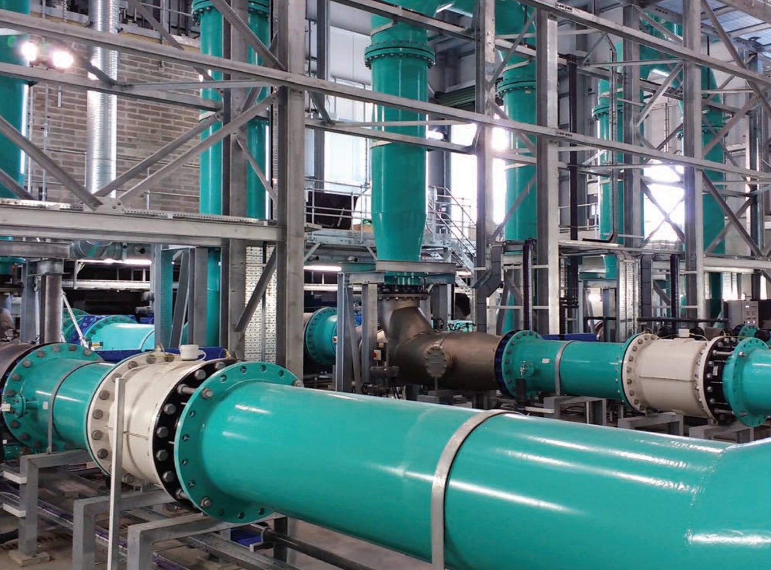
UVLX-30800-30 low pressure amalgam system in situ operating at a UK drinking water plant
