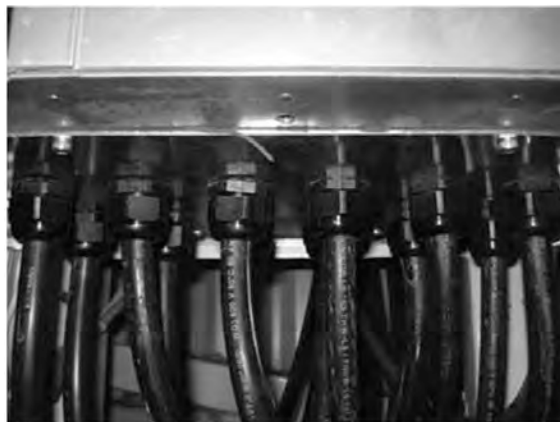
Figure 32: Example of proper installation of the connector plate
