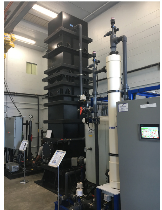
Biofiltration column from Leopold, a Xylem Brand that includes XA Underdrain and IMS 200 Media Retainer.
