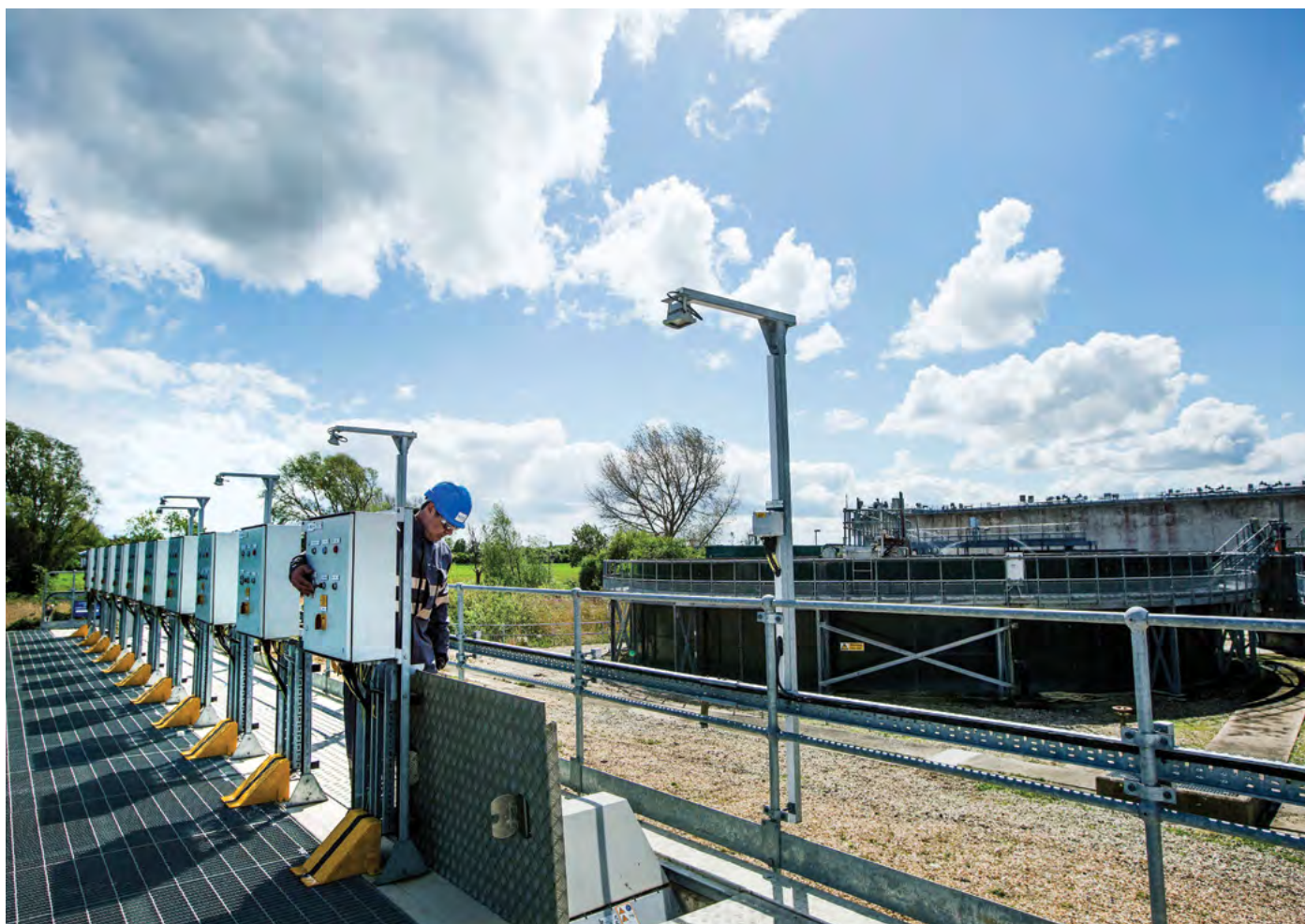
Wedeco Duron UV installation in Chichester, UK.
